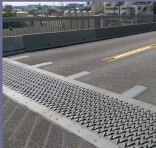
模块化模数式伸缩装置 TENSA®MODULAR expansion joint
